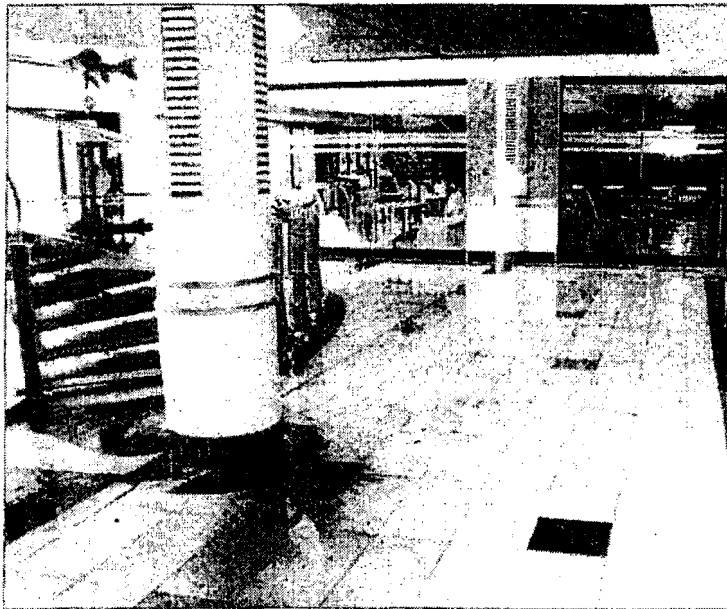
SPLASHED: Part of the Mall's flooded area.
